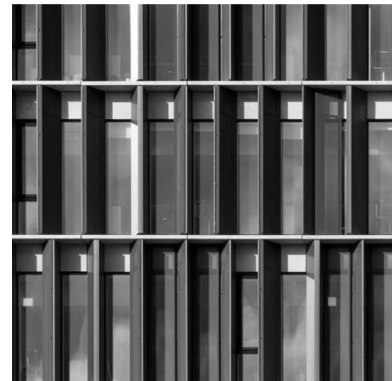
Vertical fins for solar shading
