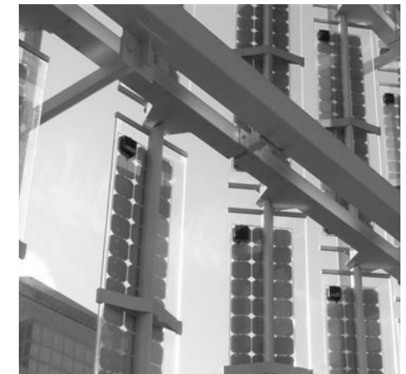
PV cells integrated into brise soleil
